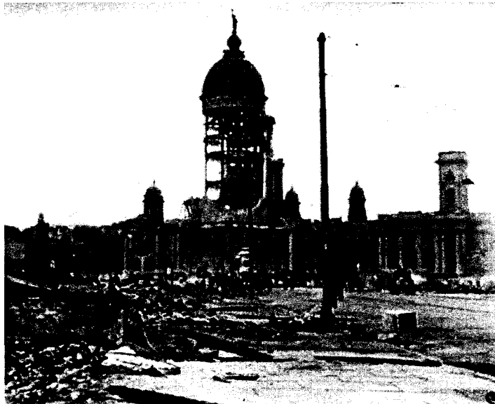
American Memory Project. Partial ruins following the 1906 San Francisco, California, earthquake. Courtesy of the Library of Congress.
