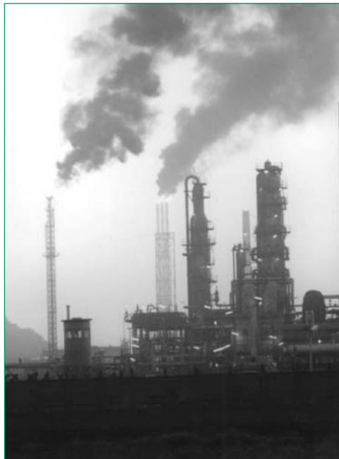
Figure 2.1: Warm air rising from SAPREF stacks, October 2002
